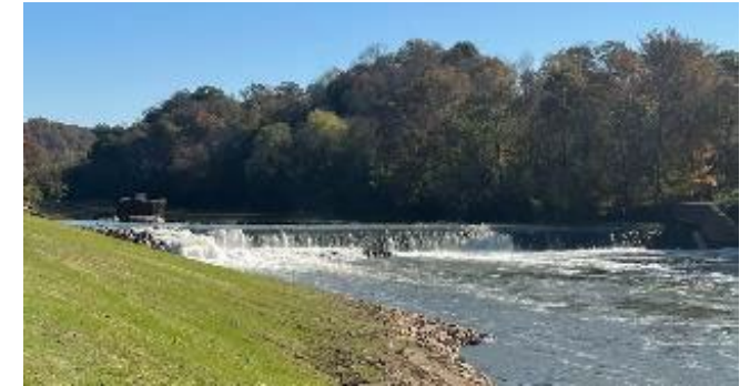
Green River Lock and Dam 5
