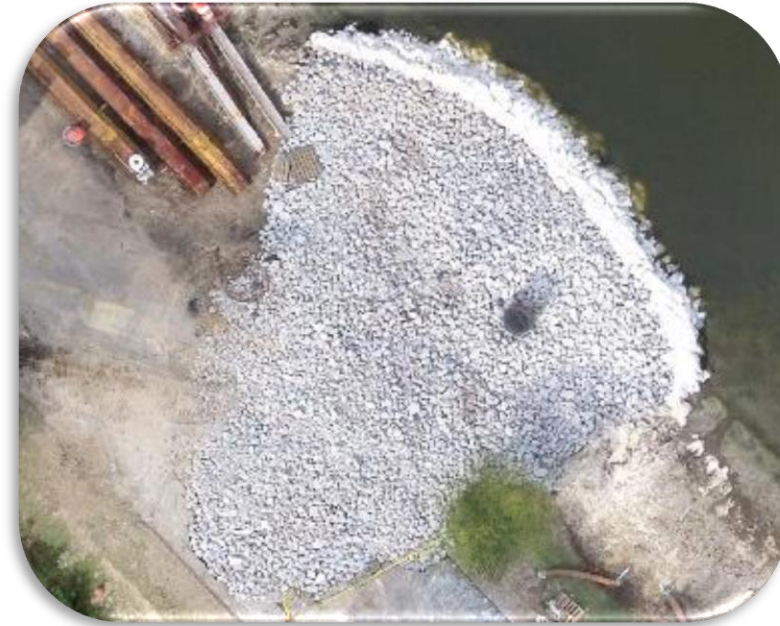
-Construction at Beaver Dam
