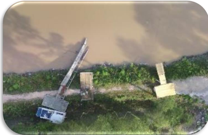
-Debris remnants from Katherine Dam overtopping
