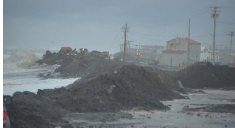
Sacrificial berm during a storm
