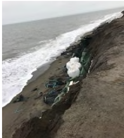
Super sacs used to protect eroding bluff
