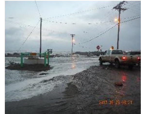
Flooding at a Utilador pump station
