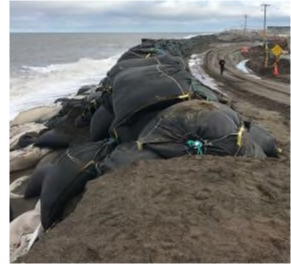
Super sac berm protecting a road
