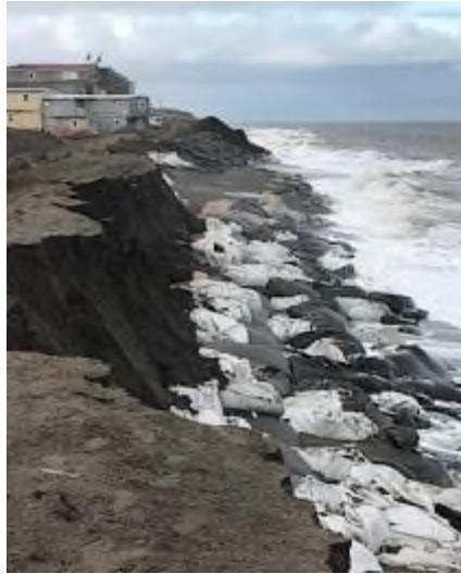
Super sacs used to protect eroding bluff
