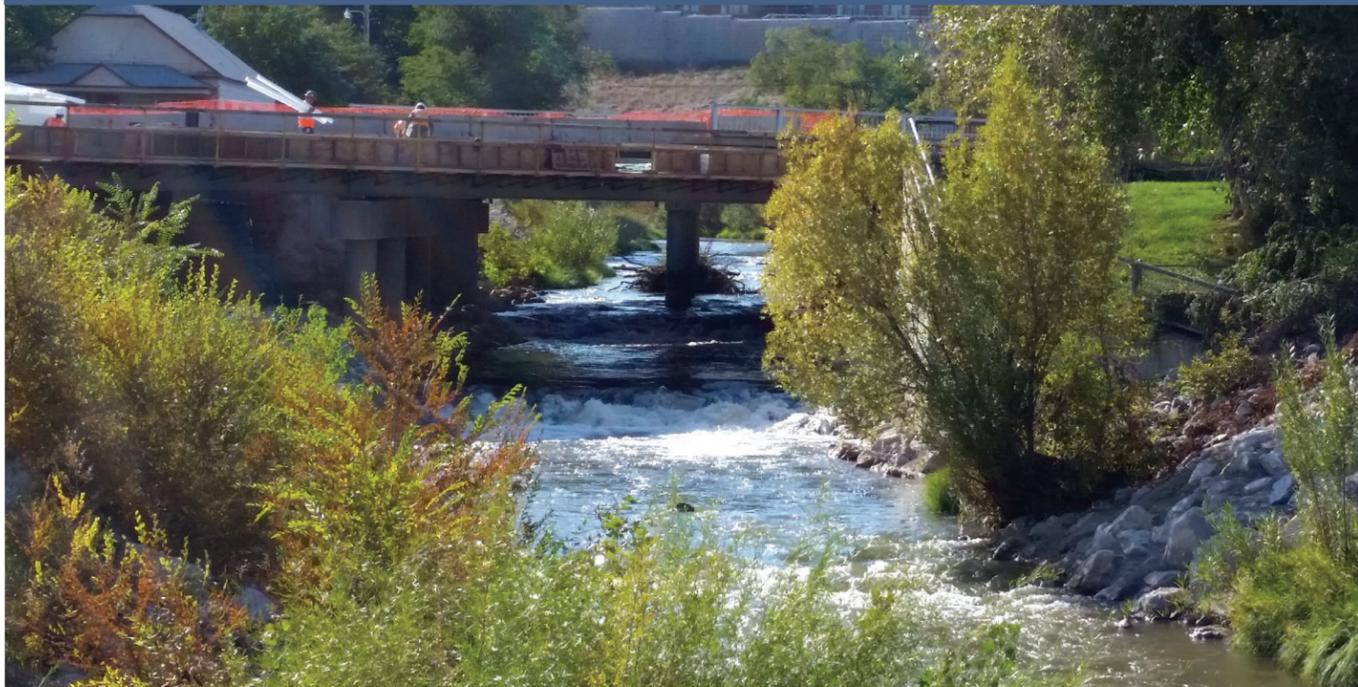
UNDER THE TENTATIVE PLAN, THE FOUR CURRENT DROP STRUCTURES ON BIG GOOSE CREEK, WHICH ARE CURRENTLY FISH PASSAGE BARRIERS, WILL BE REPLACED WITH A SERIES OF APPROXIMATELY 25 STRUCTURES SPREAD OUT FURTHER ALONG THE RIVER WITH A SMALLER VERTICAL DROP TO FACILITATE INCREASED PASSAGE FOR NATIVE COLD WATER FISH SPECIES SUCH AS THE CUTTHROAT TROUT. (SOURCE: USACE)
