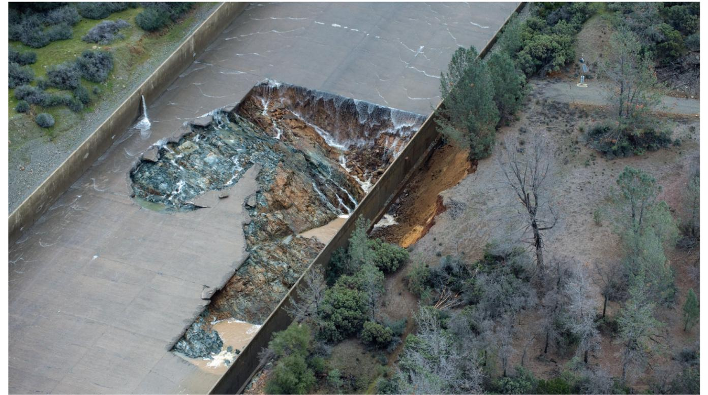
THE CALIFORNIA DEPARTMENT OF WATER RESOURCES SUSPENDED FLOWS FROM THE LAKE OROVILLE FLOOD CONTROL SPILLWAY AFTER A CONCRETE SECTION ERODED ON THE MIDDLE SECTION OF THE SPILLWAY. (SOURCE: KELLY M. GROW/CALIFORNIA DEPARTMENT OF WATER RESOURCES)
