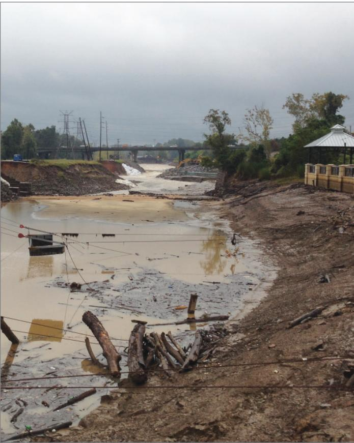
IMAGES OF THE COLUMBIA CANAL BREACH. DURING THE 2015 RAIN EVENT THE CANAL WAS FLOODED AS THE GATES TO THE BROAD RIVER (BUILT IN THE 1800S) COULD NOT BE CLOSED, RESULTING IN THE WATER TOPPING THE CANAL AND EATING THROUGH THE EMBANKMENT.
