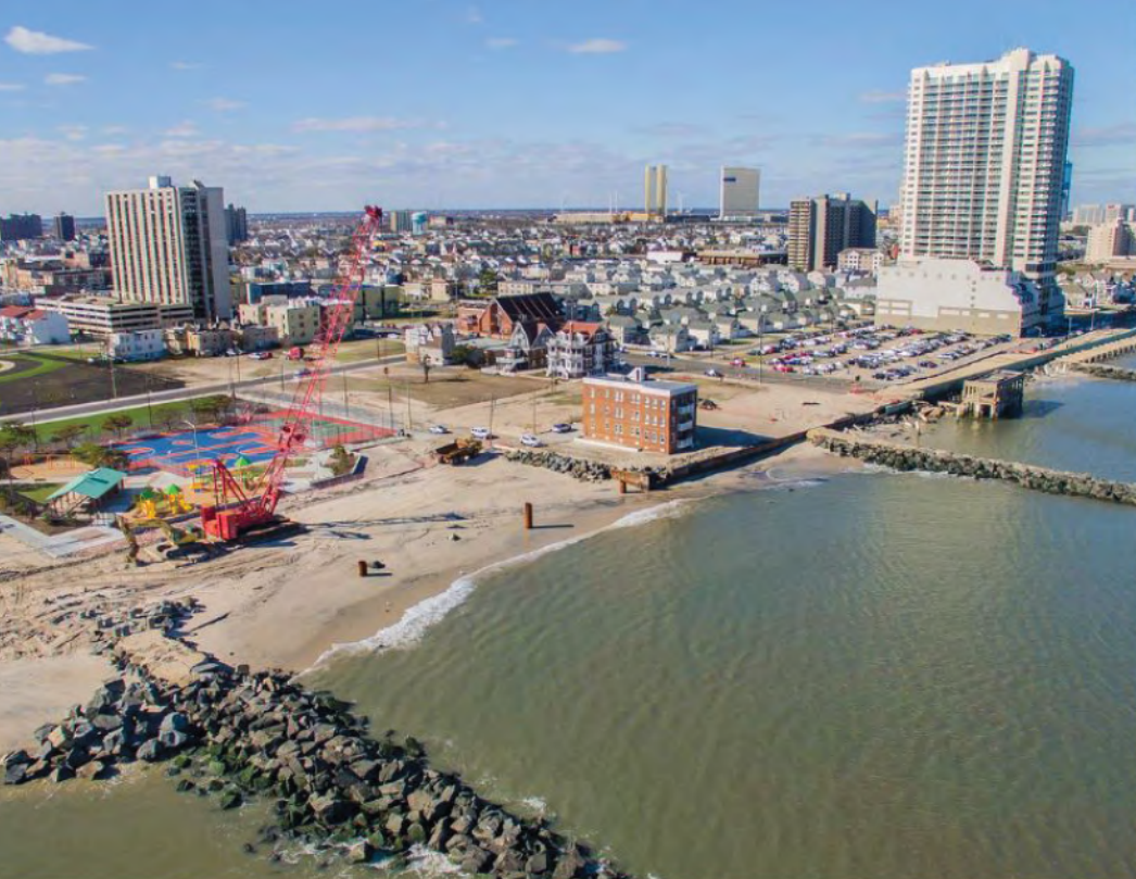
1,740 feet of seawall USACE built helps protect Atlantic City, NJ, from sea level rise and storm surge
