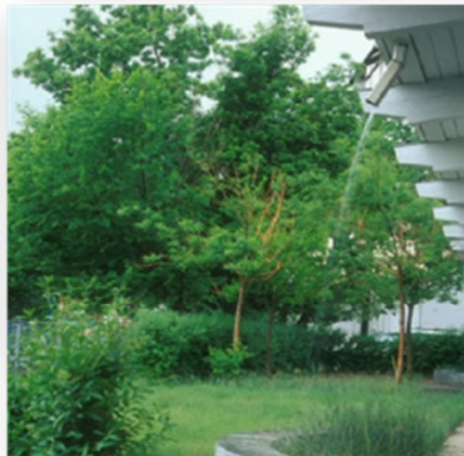
Irrigation by disconnected downspout Denver, CO
