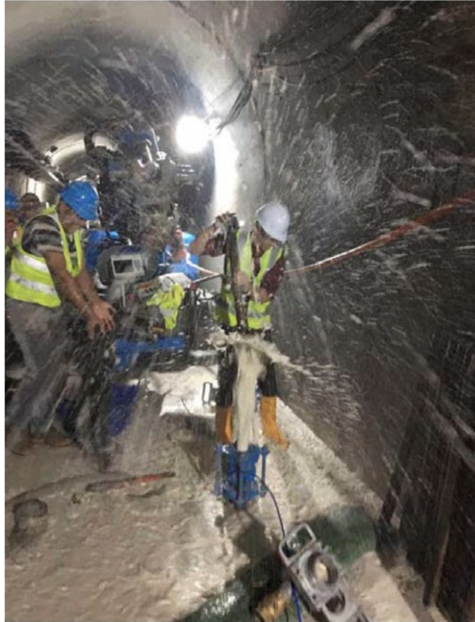
Figure 3-14. Problem Holes were Difficult to Close
